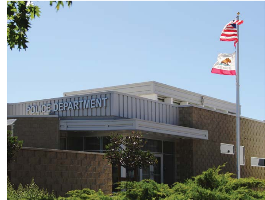
Campus Police / Central Plant
